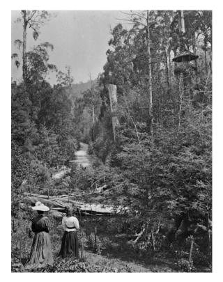
FIGURE 12 A roofed, trunk-encircling treehouse at the Hermitage (upper right). Access is by a twostage ladder and lower picketed platform to the right of the tree trunk. The women also face a log footbridge and road. Undated photo by J. W. Lindt (courtesy State Library of Victoria, H85.40/1, b48369).
